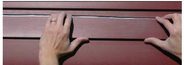
**NOTE:** Cut through any double sided tape if necessary. Be sure not to damage the house wrap underneath. Any damage that occurs to the house wrap during the replacement process must be repaired before the replacement piece is installed.
